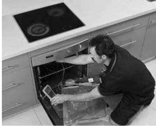
Installed electrical cooker
