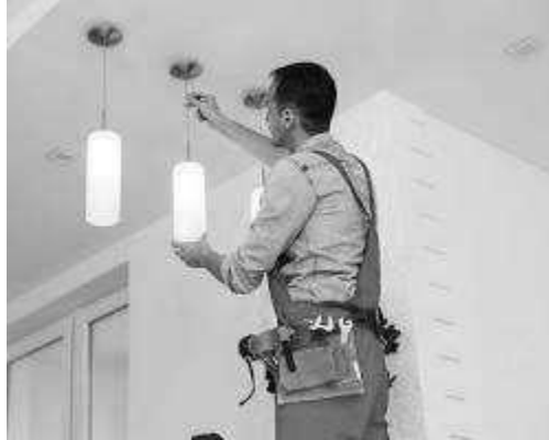
Installed light fixture
